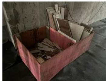
Figure 2: Construction waste segregated at the construction site. Source: Author, 2024.
