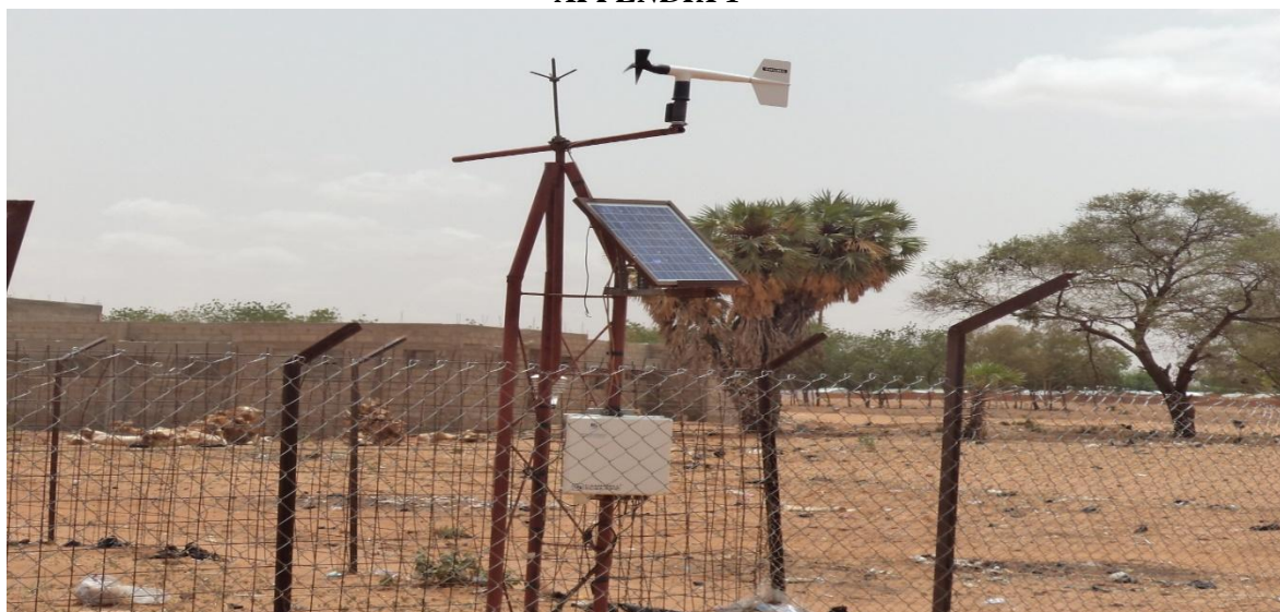
Figure A: Picture of the weather station installed at mini market of UDUS, Main Campus, December, 2016.
