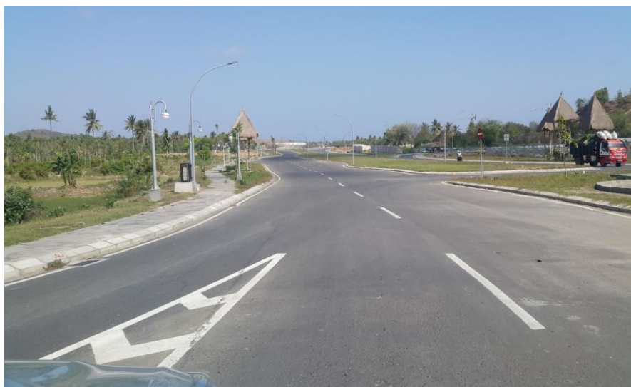
Fig. 2. Development of infrastructure to support KEK Mandalika
