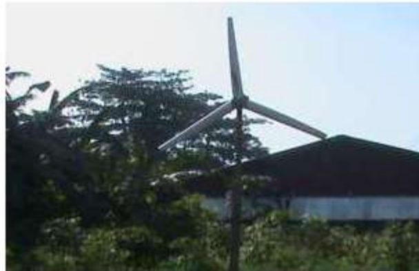
Figure 8 Wind Power Plant
