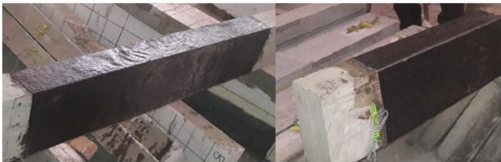
Fig.(10)Placing carbon fiber in strengthening zones
