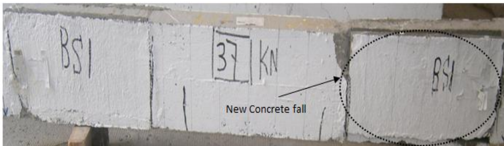
Fig.(26) Crack pattern after failure – BS1
