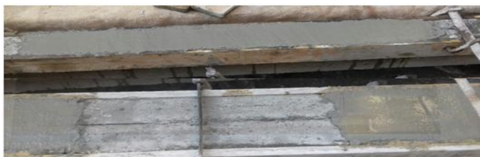
Fig.(6) Casting new concrete mixture in strengthening zones
