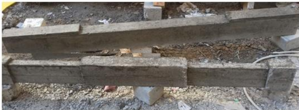
Fig.(4) Preparation a groove in strengthening zones
