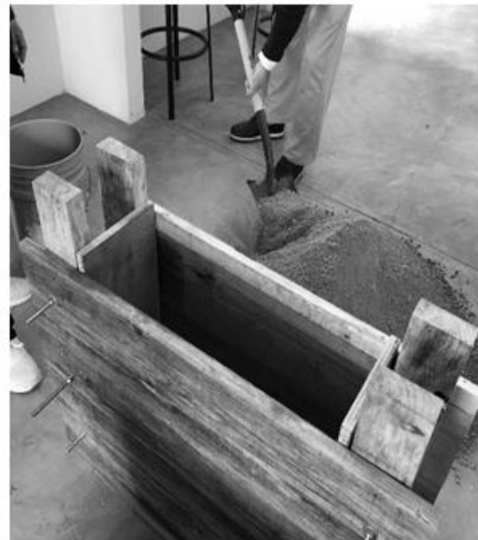
Images 1 and 2. Soil screening, mixing and colocation in the formwork for later tamping. Photo: Gloria Esmeralda del Ángel Cavazos. Architect.
