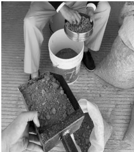
Images 1 and 2. Soil screening, mixing and colocation in the formwork for later tamping. Photo: Gloria Esmeralda del Ángel Cavazos. Architect.
