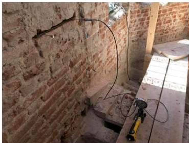
Figure 7. The mechanical tests: Single flat-jack test
