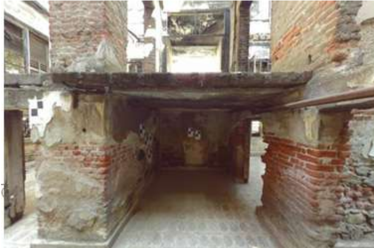
Figure 5. The reinforced concrete slab in the entrance part of the building
