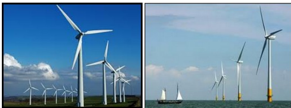
Figure 1: Wind farms on land and Offshore
