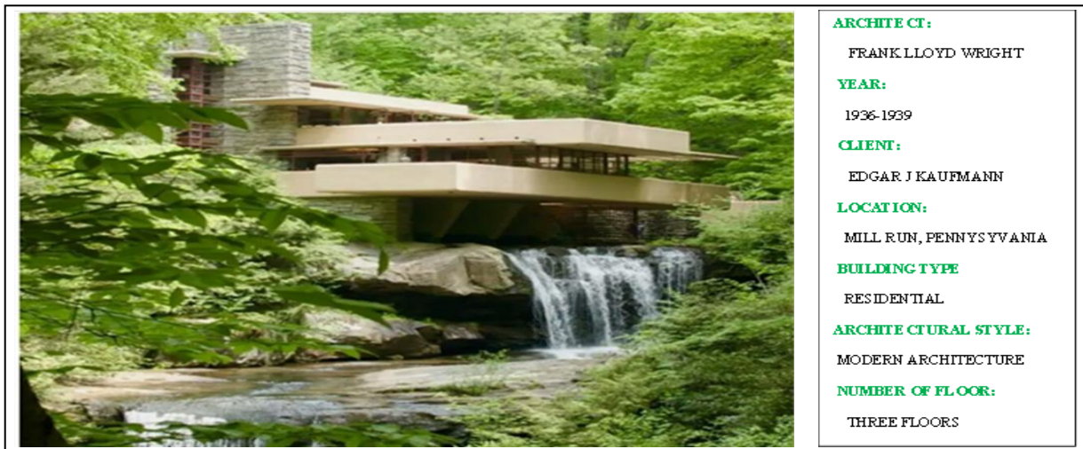
Figure 3.1 FRANK LLOYD WRIGHT FALLING WATERS
