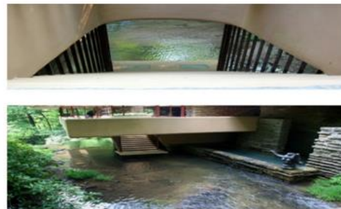
Figure 3.7 Stair hall, Exterior view
