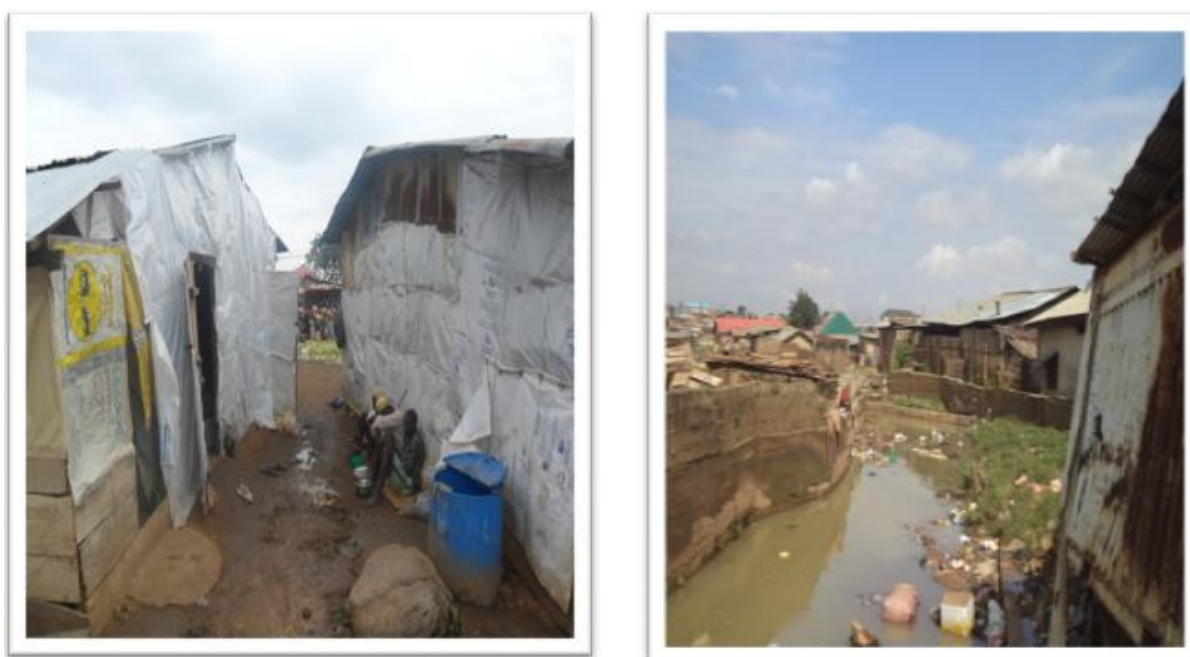
Plate 1: Poor Housing and Environmental Condition in Mararaba
