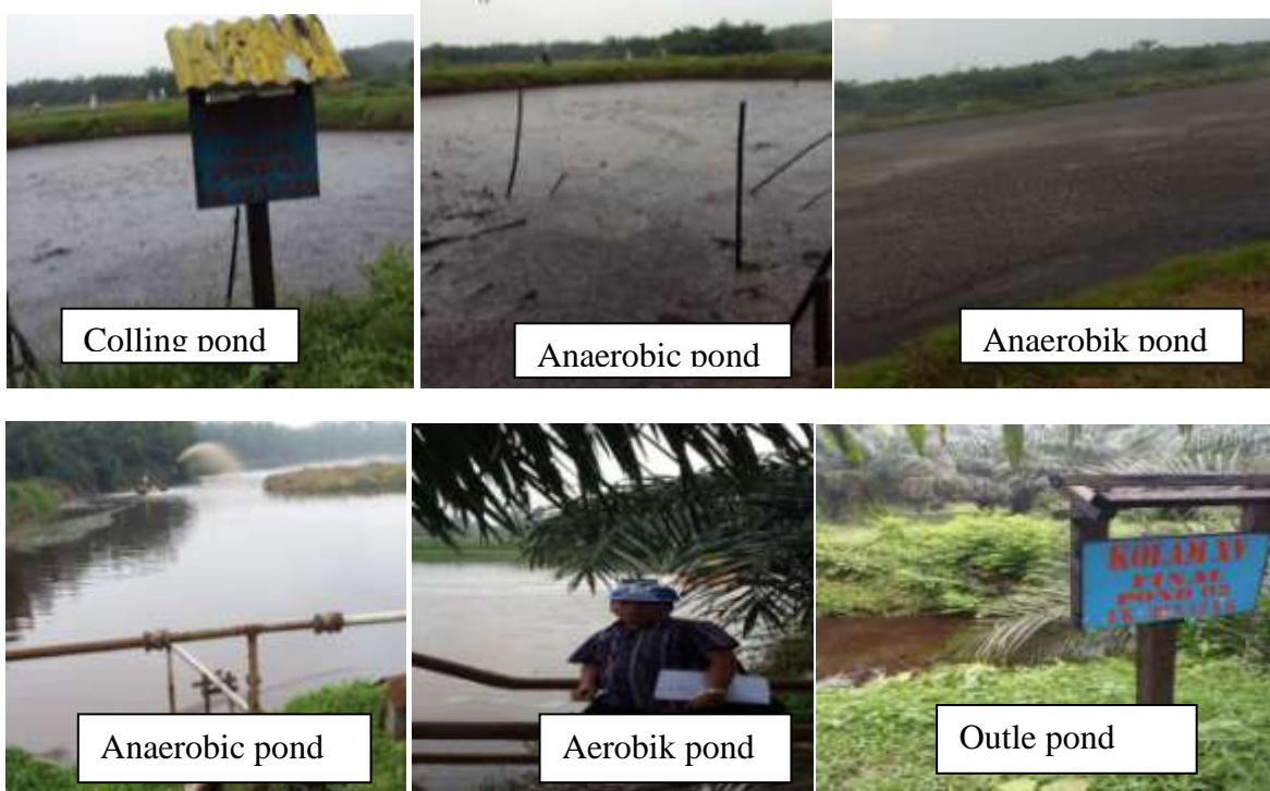
Picture 2.Foto WWTP Pools Palm Oil Factory DM Company Jambi Indonesia
