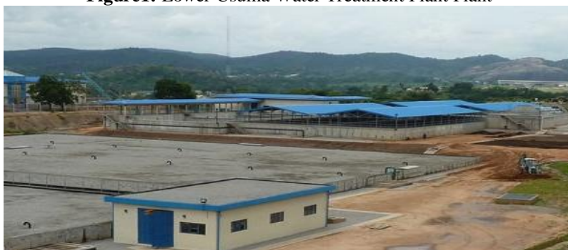
Figure1: Lower Usuma Water Treatment Plant Plant
