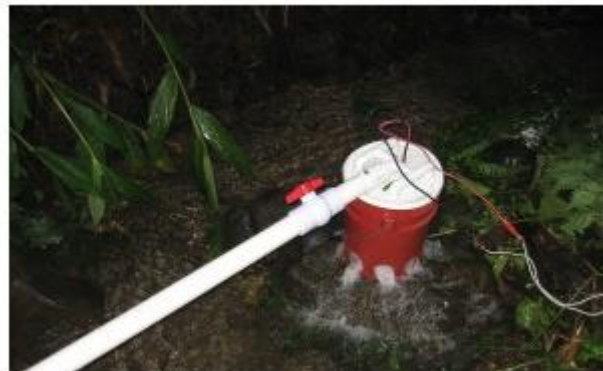
Fig. 2 Generator and Penstock at La Florida
