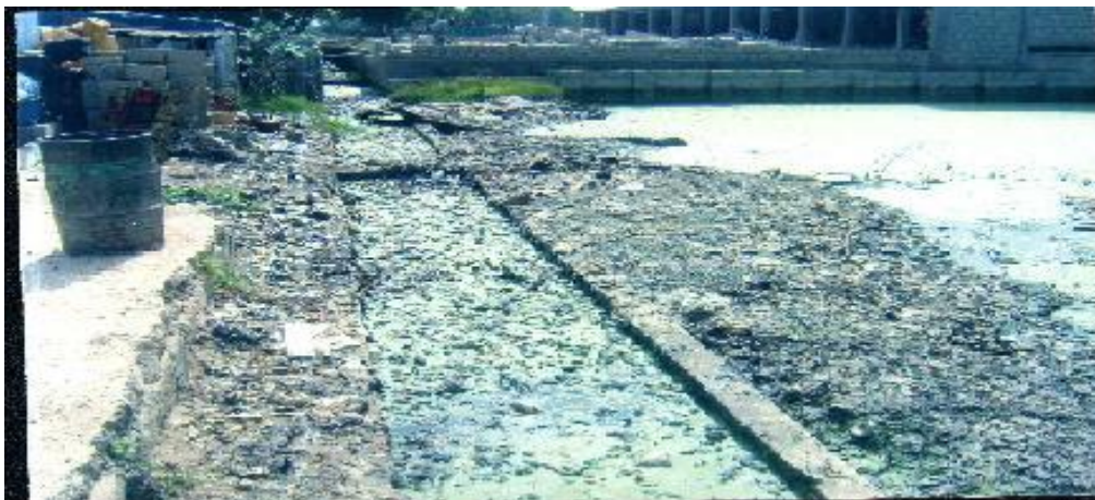
Plate 3: Drainage filled with Garbage in Ngomari Ward in Maiduguri
