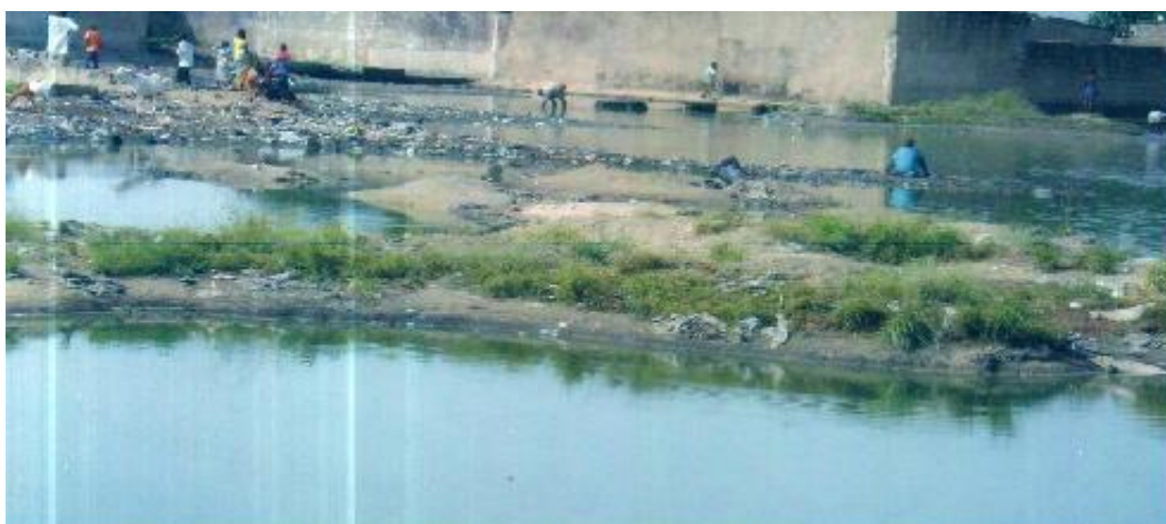
Plate 4: Sand Filling Process (Reclamation) in Moduganari Ward in Maiduguri
