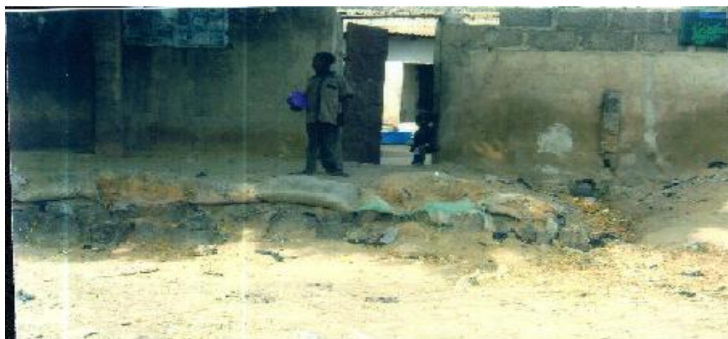
Plate 5: Sand Bagging to Prevent Flood entering a House in Mashimari Ward in Maiduguri
