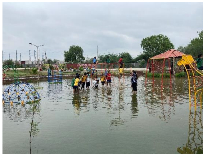
Rainwater accumulation during monsoon session at Hostel campus
