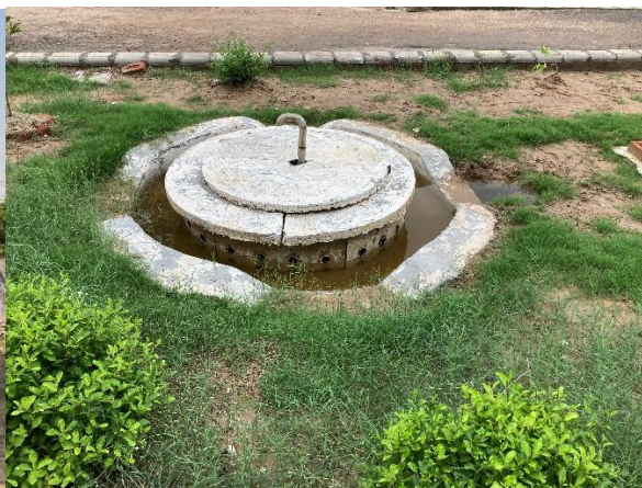
Rainwater discharge well
