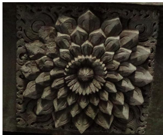
Photograph-4: Lotus on Upper portion of Beam
