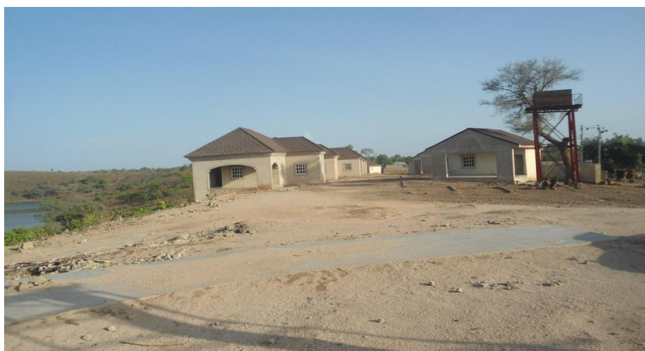
Plate.2: Guest House under Rehabilitation and construction in Tilla Crater Lake
