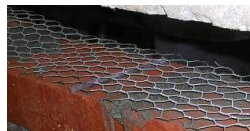
Fig 1: Mesh bands along bed joints
