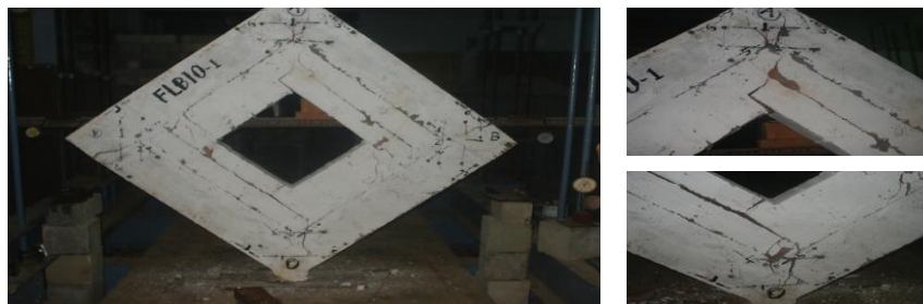
Fig 13: Failure pattern of infilled frame with central opening (FLBIO)
