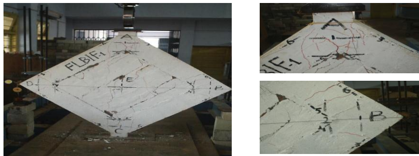
Fig 12: Failure pattern of infilled frame with ferrocement bands (FLBIF)
