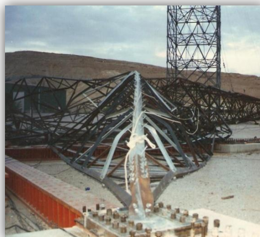
Fig. (4) Assumption: (T1) second failure (Destruction Test)
