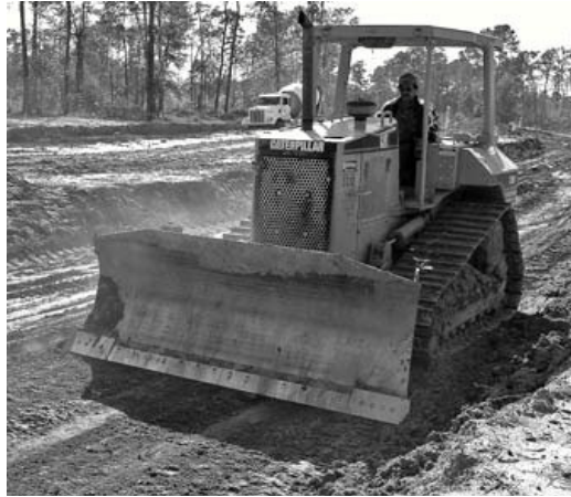
Fig 7: excavation of surface soil
