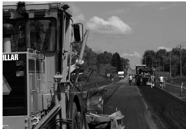
Fig 1: laying of pavement by soil stabilization process
