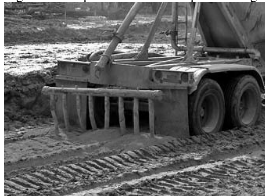
Fig 9: mixing of fly ash with soil
