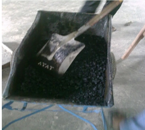
Fig 4: bitumen mixed with aggregate
