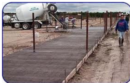
Fig 12: preparation of layer for curing
