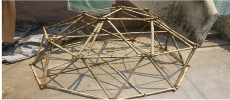
Fig 2.1 Dome construction at initial stage
