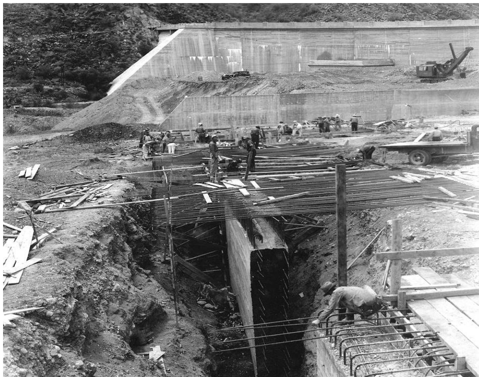
Figure-5 Picture Taken During Construction
