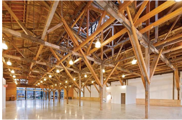
Figure 5: Use of ltimbers for structural framework.
