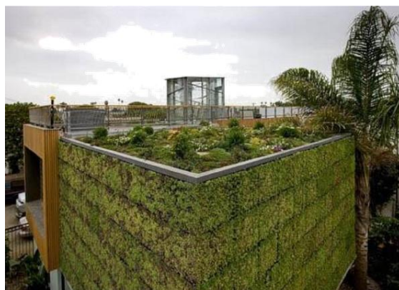
Figure 9: Green walls with green roof
