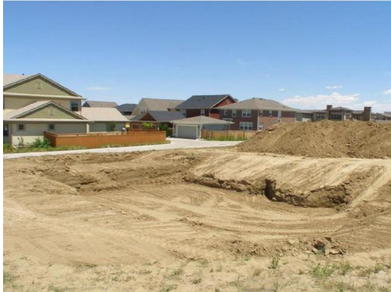
Figure 1: Soil arrangements on site
