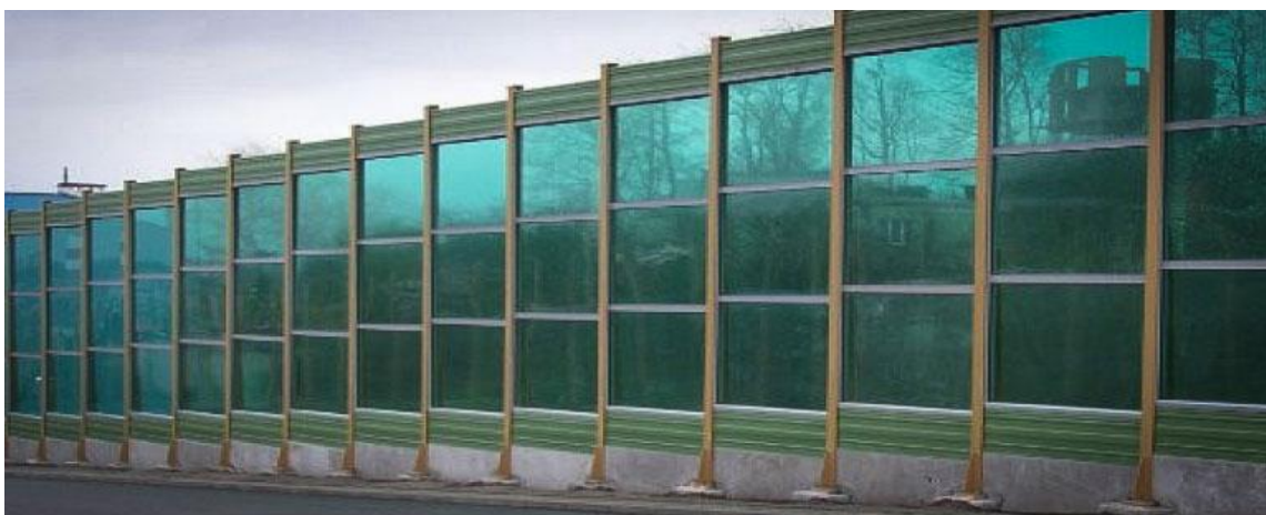
Fig 6.1: Noise barriers oriented at an angle ( www.noisebarriers-hosekra.com )
