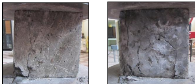
Fig 13 Whitish Appearance on Specimens after Sulphuric Acid Curing
