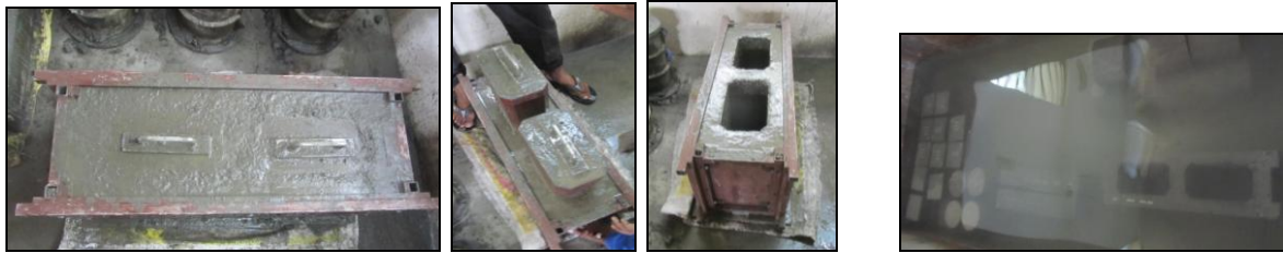
Fig 6 Casting and Curing of Designed Hollow Block
