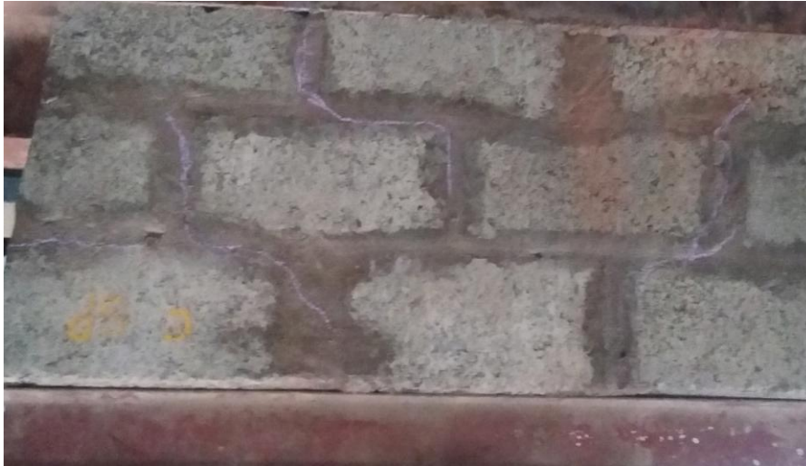
Fig5: Failure pattern of flyash block wall
