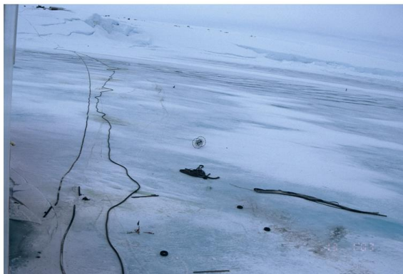
Fig.1. Transfer of fuel through flexible pipes over sea-ice.
