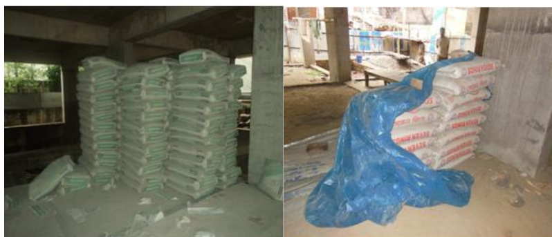
Figure 1: Typical storing of cement at site.
