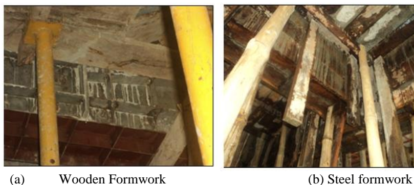
Figure 8: Typical formwork used at site
