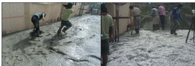
Figure 5: Slab casting by ready mixed concrete
