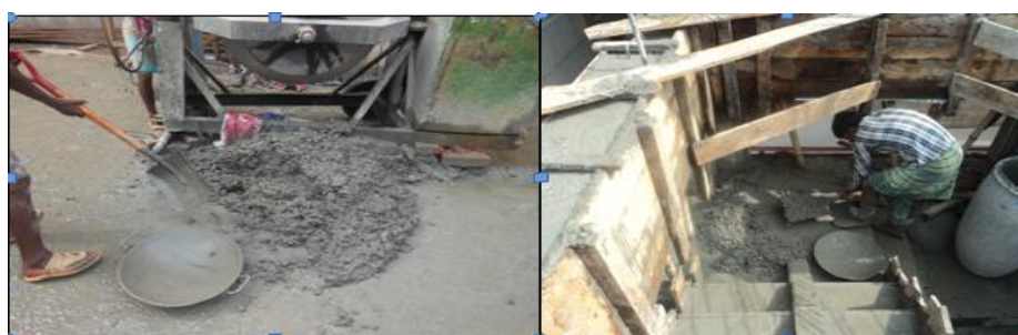
Figure 6: Slab casting by in situ concrete
