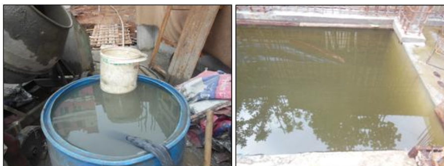
Figure 4: Water used for concreting
