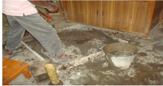
Figure 2.3 Shows the mixing of concrete
