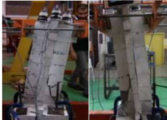
Figure 14: Crushed at 3rd, 4th Blocks and of Last Block In front and Rear View of Model 2 Failure
