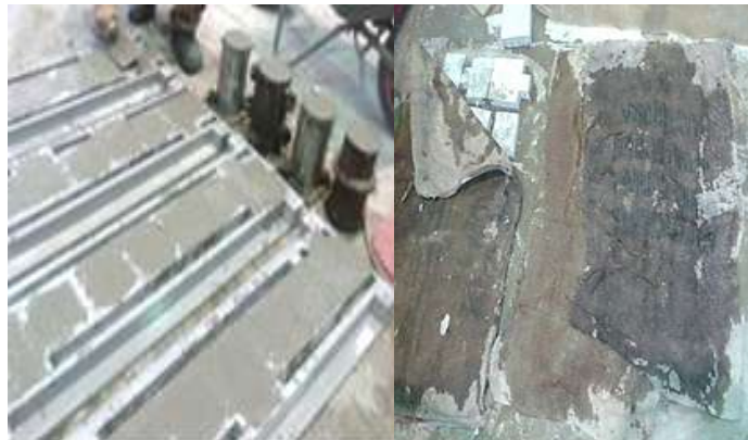
Figure 4: Casting and curing works
