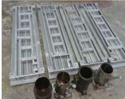
Figure 3: Formwork and Reinforcement Preparation
