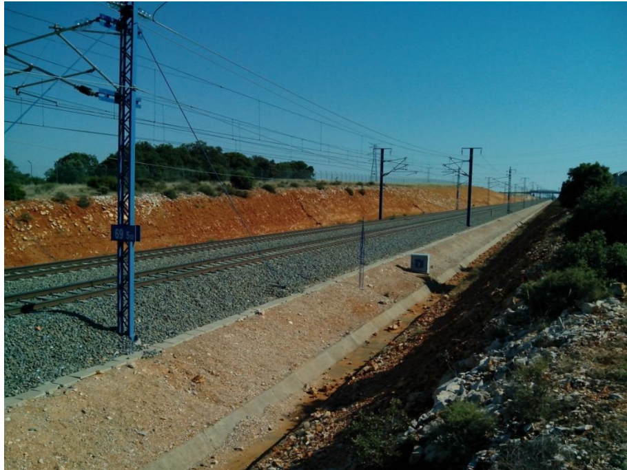
Fig.1. Monitored track section in the high speed line Madrid-Barcelona-French Border
