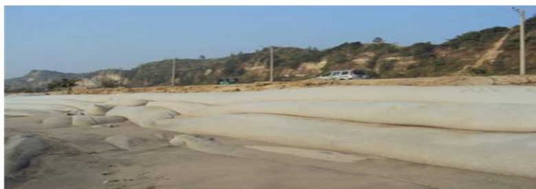
Fig 2: Hill side protection with jute geotextile
