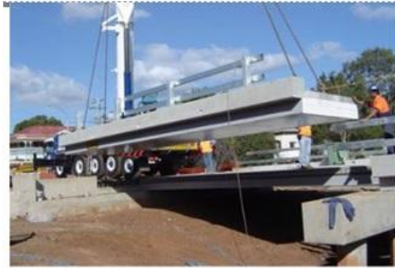
(b) Taromeo Creek Bridge
