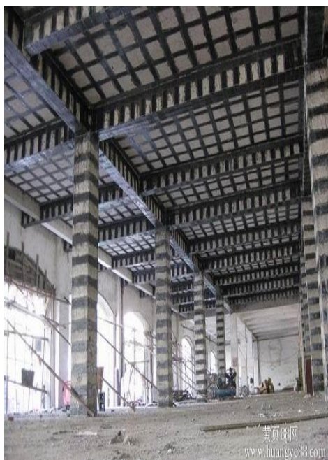
Figure 4: Bidirectional/Unidirectional/Mixed Knitted/Construction reinforcement carbon fiber fabrics
