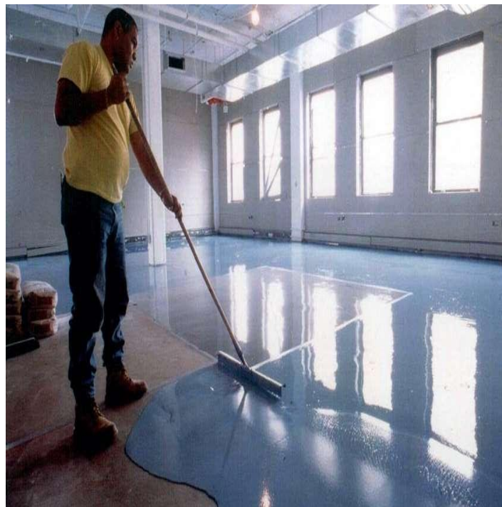
Figure 6: Seamless Epoxy Floor Resurfacer Covers Damaged Floors
