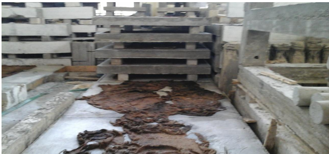
Fig. (8) Curing of Flat Slab Concrete Specimens
