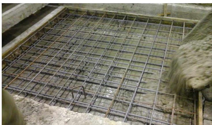
Figure (7) Pouring Concrete of Flat Slab Specimen.
