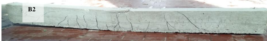
Figure 4: Crack pattern of MK_1S_1A_1C_1B
