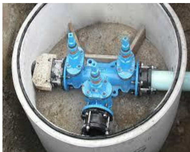
Fig.2.5. Sluice valve repair
