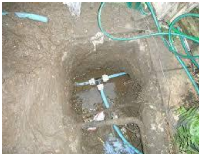
Fig.2.6. Main repaired connections
