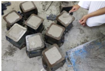
Fig.8 Casting of GPC Cubes
