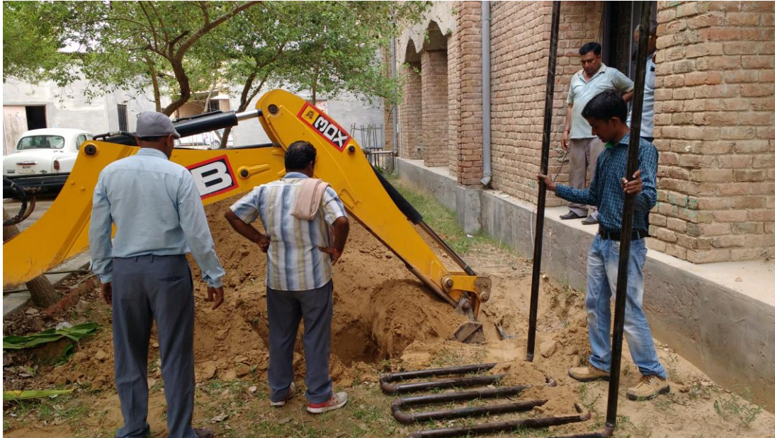
Fig. 6: Installation of setup using JCB machine
