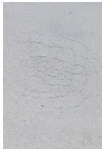
Fig.3 Fatigue Cracking
