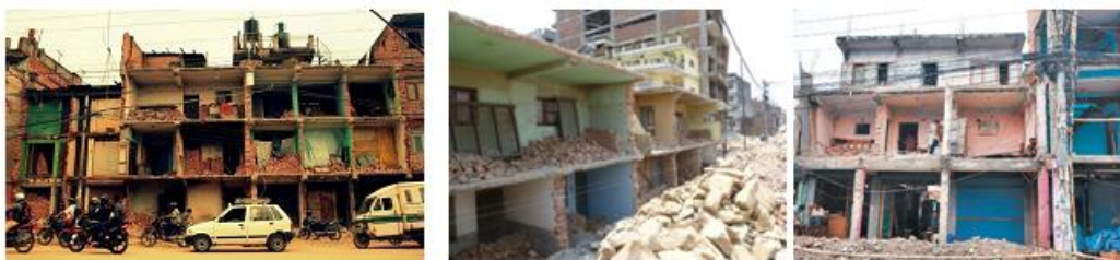
Figure 1: Dismantled buildings during Road Widening Project in Kathmandu.
