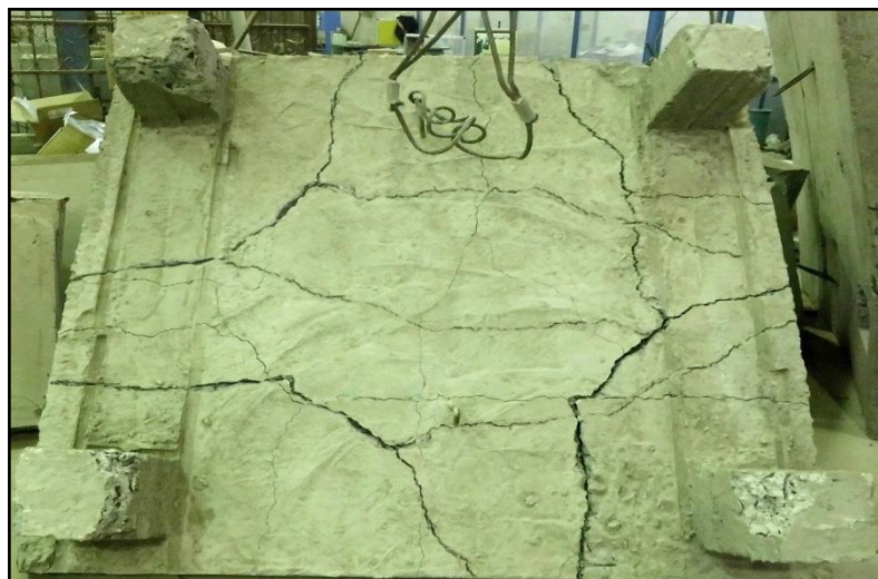
Fig.9 Crack pattern of Specimen SS
