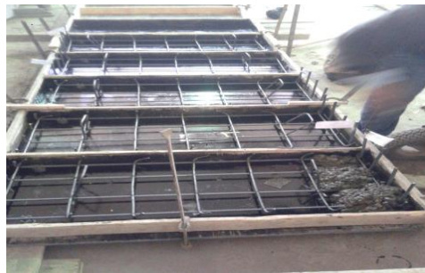
Figure (1). Steel reinforcement arrangement in wooden form.
