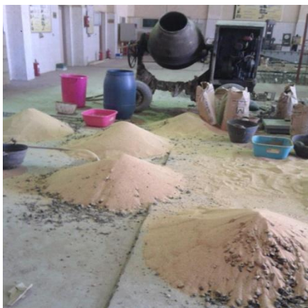
Figure (2). a. Preparing of the concrete mix ingredients.
