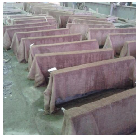
Figure (2). d. Curing of slabs.
