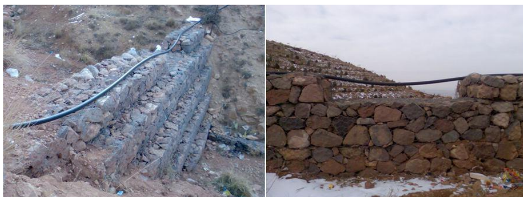
photo.2 "Gabion stepped spillway used to reduce water velocity and to collect sediments in mountain valley (left), and gabion structure in a retaining wall for slope stability (right) on Onebne-Ali mountain, north of Tabriz (IRAN) "
