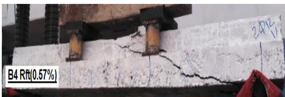
Figure (11): Crack pattern for control beam (B4)
