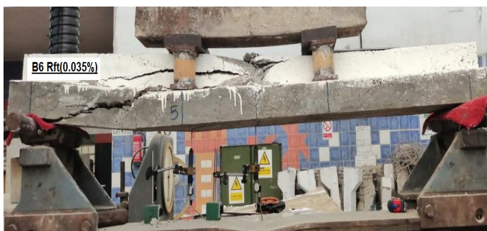
Figure (13): Crack pattern for control beam (B6)
