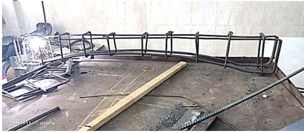
Fig.(2)Reinforcement for specimens
