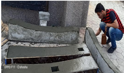
Fig.(4)concrete mixing and casting
