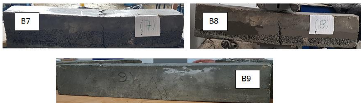
Fig. 9 Crack pattern for the tested beams
