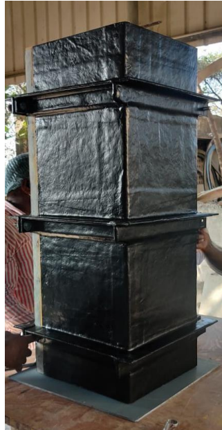
Figure 6 Completed GRP Panels with Finished Bolted ends
