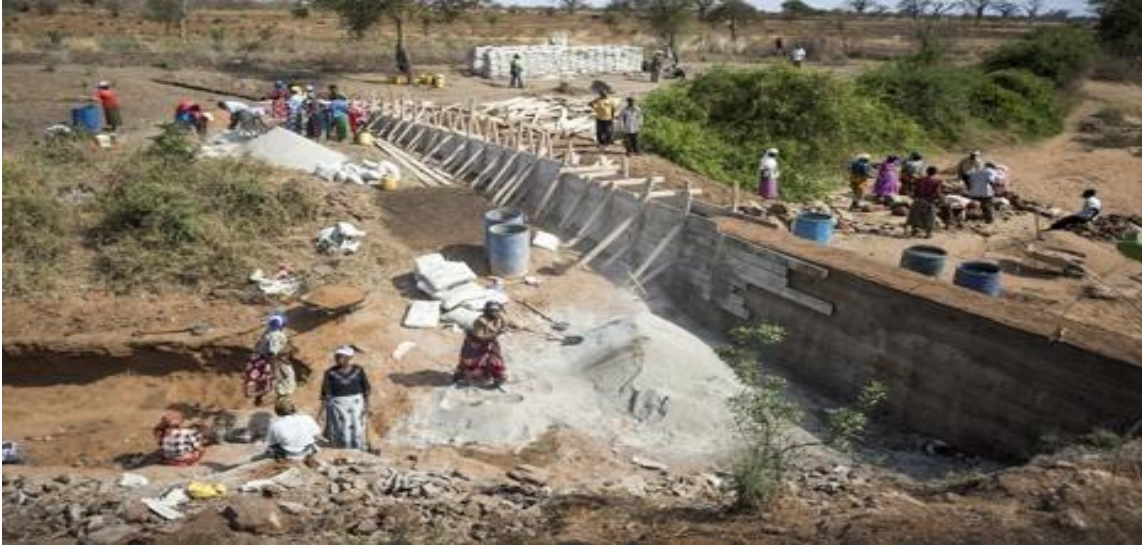
Plate 1.1: Small dams collect sand, which acts as a resilient store of water even when seasonal rains not available
