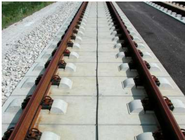
Figure 1 Ballast less track
