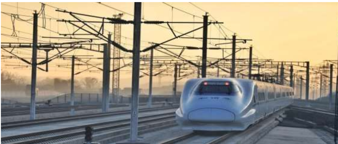
Figure 5 High speed train on ballast less track
