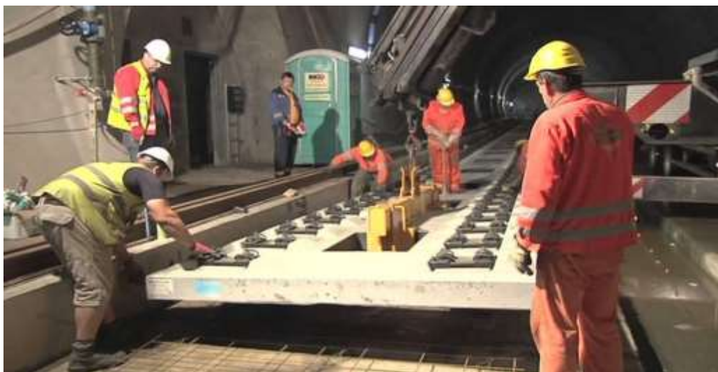
Figure 8 Application of ÖBB-PORR System
